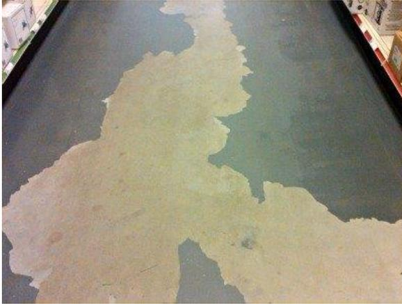
**WITHOUT A VAPOR BARRIER** to block moisture from below, the concrete floor is basically an open "sponge" that can cause problems for coatings, adhesives, and flooring materials. If an impermeable coating or flooring material is installed on top of the concrete floor, the moisture will build up below the coating and eventually cause it to blister and delaminate.
