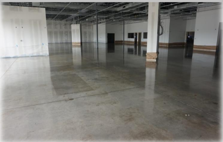
Clear Over Prepared Concrete
